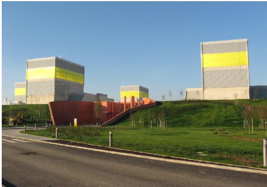
The artificial hill and the ventilation towers
